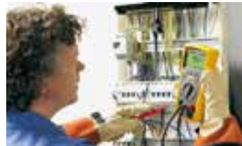
Insulation test at a distribution panel
