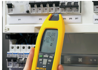
Location of fuses/breakers and assignment to circuits
